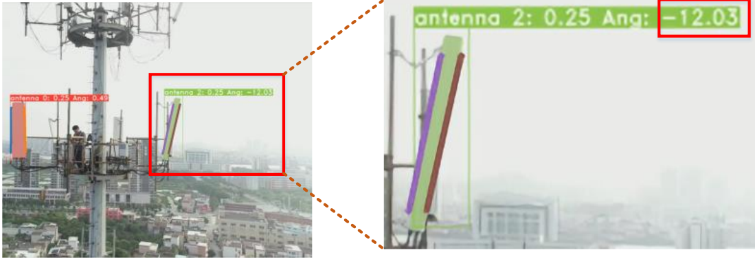
Fig. 7. Fitting pixel coordinates of the mask edge to calculate the antennas down-tilt angle.
